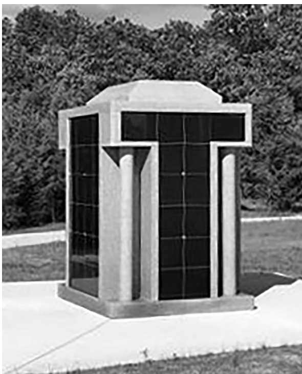
The new columbarium in St. Anthony Cemetery in Camdenon contains niches for the cremated remains of 124 people.
